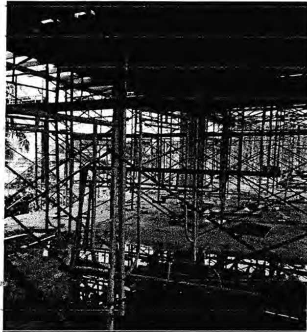
Gambar 3.5.7 Bekisting plat lantai
