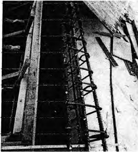
Gambar 3.5.7 Bekisting balok
