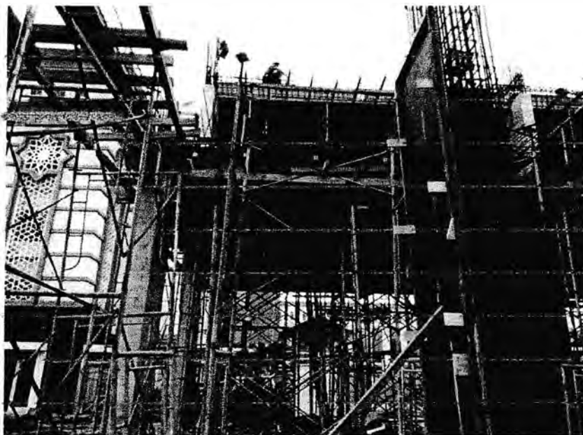
Gambar 3.5.7 Bekisting kolom
