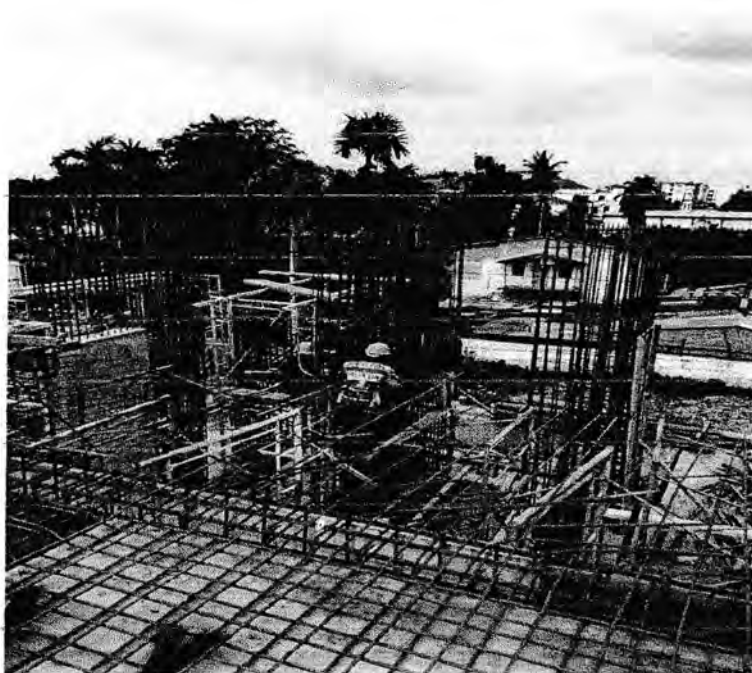
Gambar. Making Kolom
