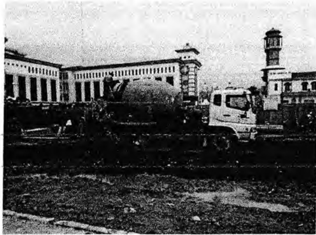
Gambar 3.1.2 Beton ready mix
