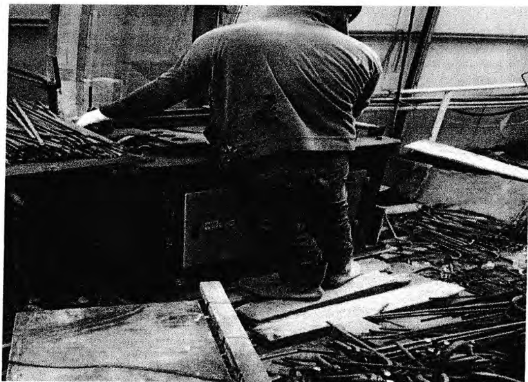
Gambar 3.5 Bar Bending
