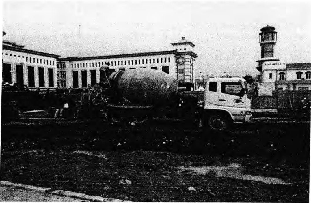
Gambar 3.2 Beton ready mix
