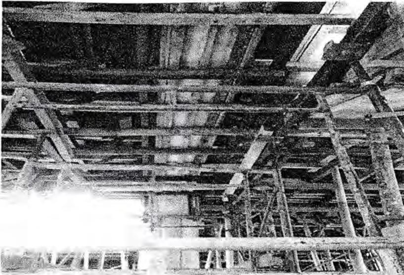
Gambar 3.23. Bekisting balok
