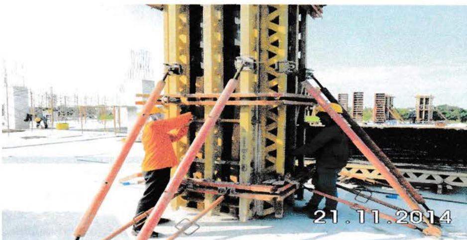
**Gambar 3.1. Bekisting kolom**
