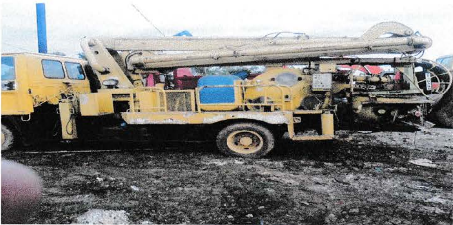
Gambar ; Pump Concrete
