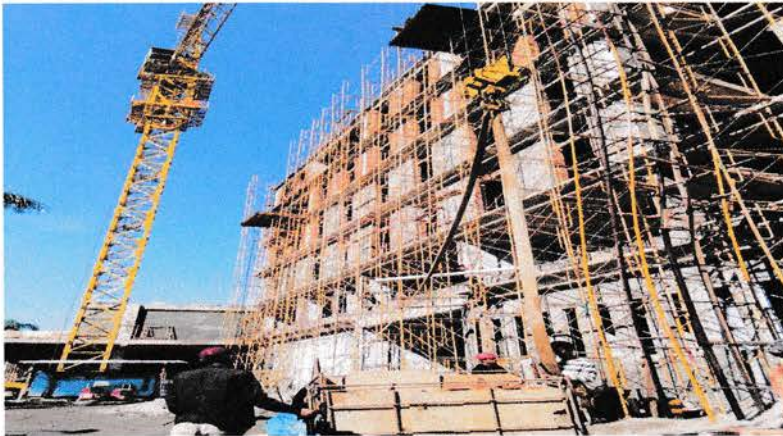
Gambar : Tower Crane
