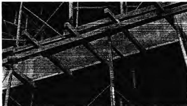
Gambar 3.14 Bekisting Balok
