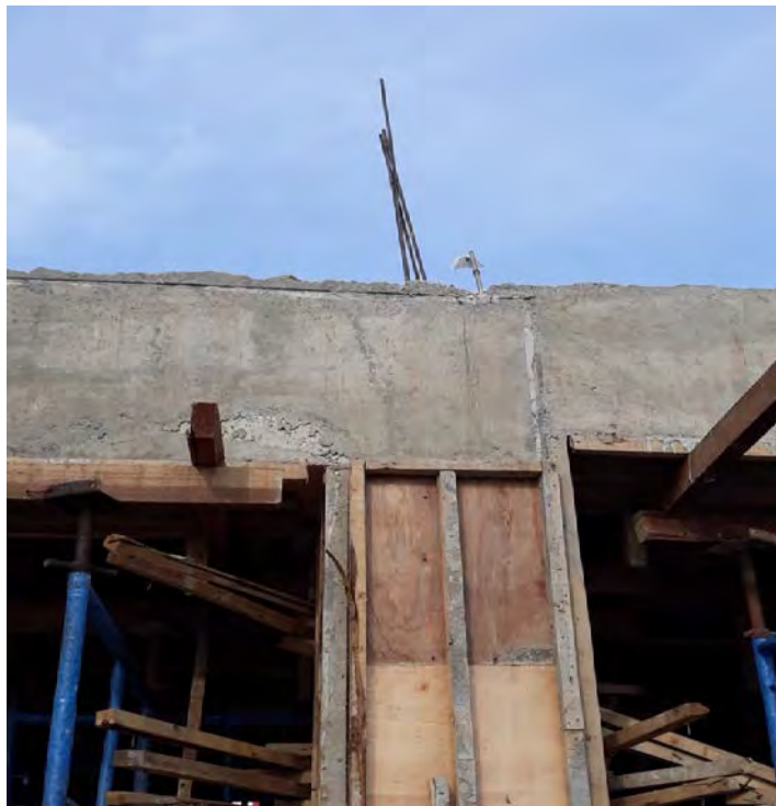
Gambar 3.19 Bekisting balok
