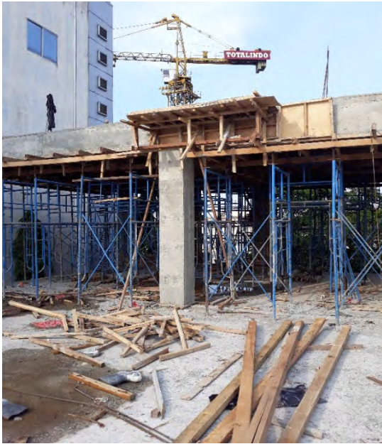
Gambar 1.1 Bekisting Balok
