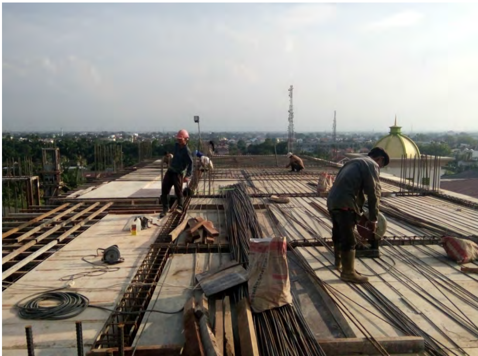
Gambar 3.20 Bekisting plat lantai
