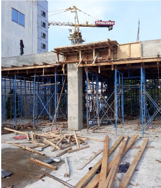
Gambar 1.1 Bekisting Balok
