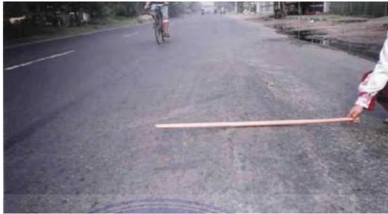
Gambar 32. Retak susut (Shahin 2003)
