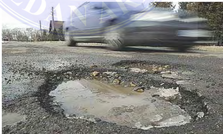
Gambar 39. Lubang, (Carro 2011)
