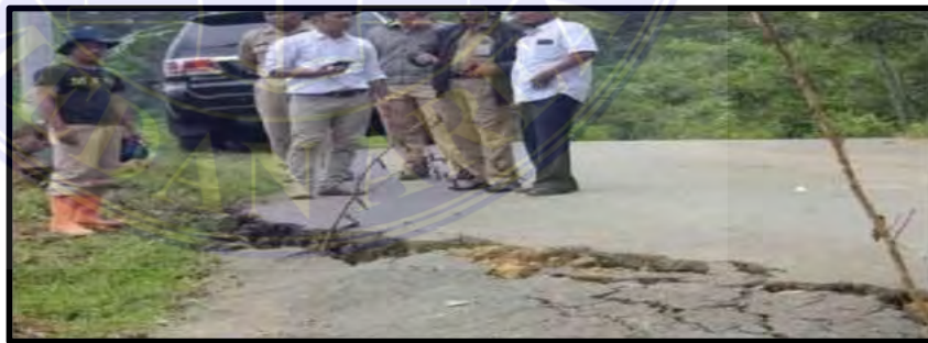
Gambar 15. Amblas ( grade depressions ) ( https://dpu.kulonprogokab.go.id )
