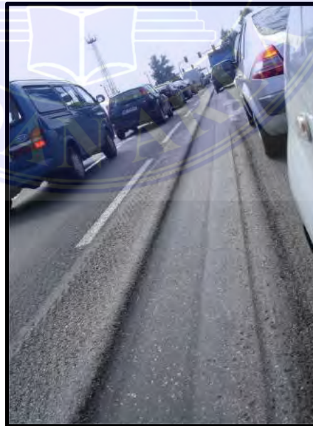
Gambar 12. Alur ( ruts ) ( https://en.wikipedia.org/wiki/Rut_%28roads%29 )
