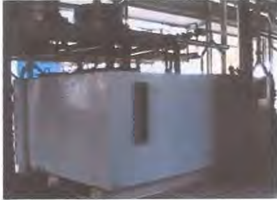
Gambar 3.13. Crude oil Tank
