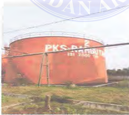
Gambar 3. 29 Oil Storage Tank
