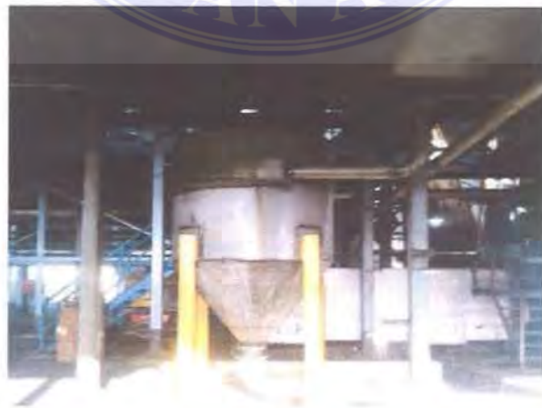
Gambar 3.17 Sand Trap Tank
