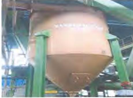
**Gambar 6. *Sand Trap Tank***
