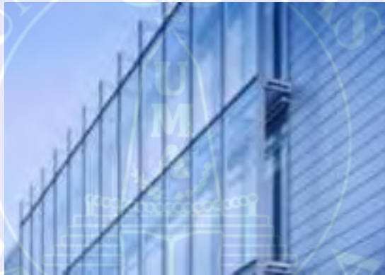
Gambar 5.2. Sistem Curtain Wall
