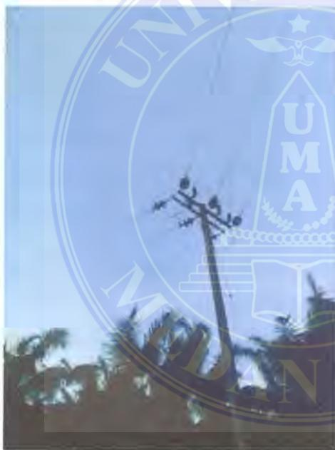
Gambar 2.7.3 Double Support on Single/ Double Pole (Type A 3)
