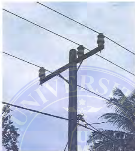
Gambar 2.8 Single support on single pole ( Tipe A1)
