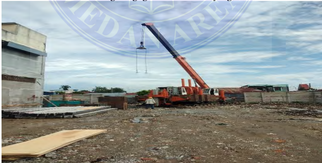
Gambar 3.21 Hydraulic System (Hydraulic Press-in) Sumber Data : Lapangan
