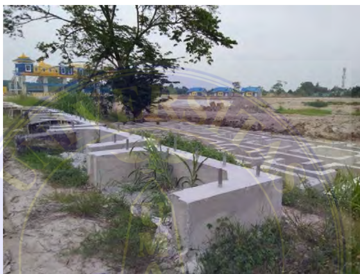
Gambar 3.4 Box Culvert
