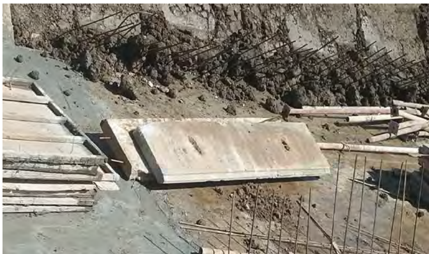
Gambar 3.5 Panel Dinding (Precast)
