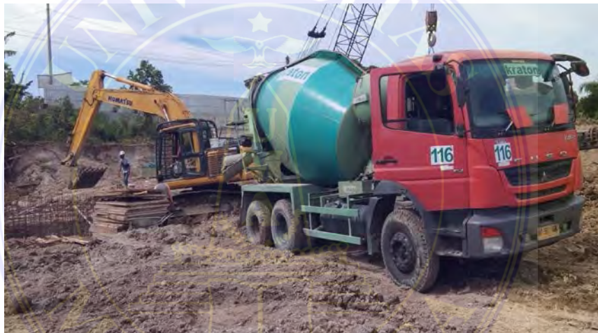
Gambar 3.1 Beton Ready Mix
