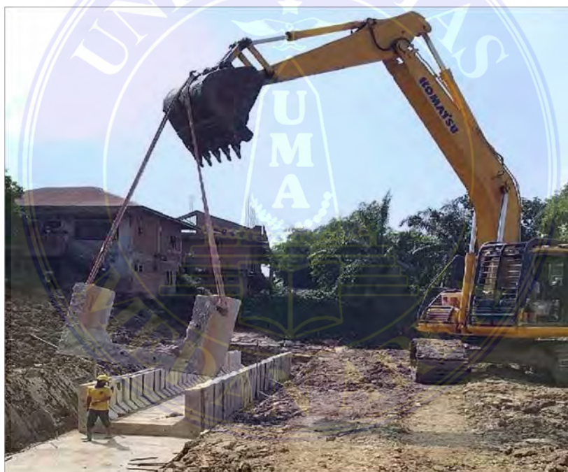
Gambar 3.12 Box Culvert
