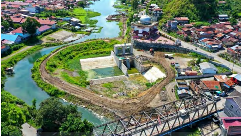
Gambar 3. 3 Regulating weir (upstream)
