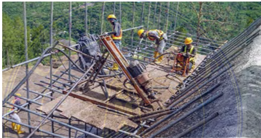
Gambar 4. 24 Drilling of Rockbolt
