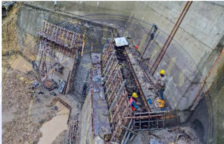
Gambar 4. 11 Formwork/Bekisting
