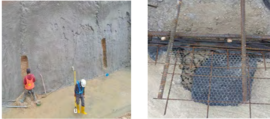
Gambar 4. 9 Gravel Drain
