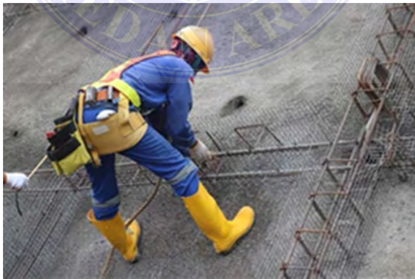
Gambar 4. 28 Bekisting free frame .
