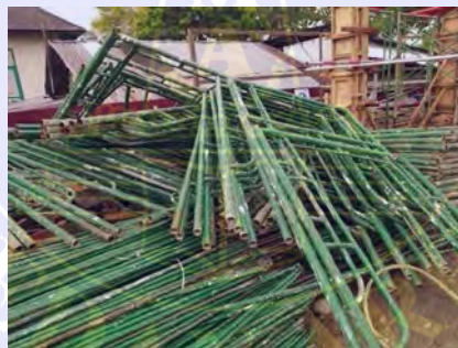
Gambar 3. 33 Perancah/ Scaffolding Sumber : Data Lapangan
