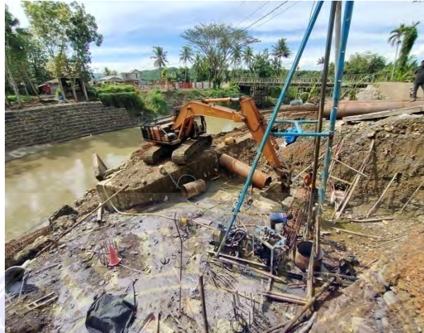
Gambar 3.3. Bore pile Machine
