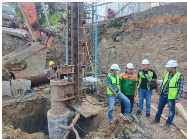
Gambar 3. Hammer PDA Test
