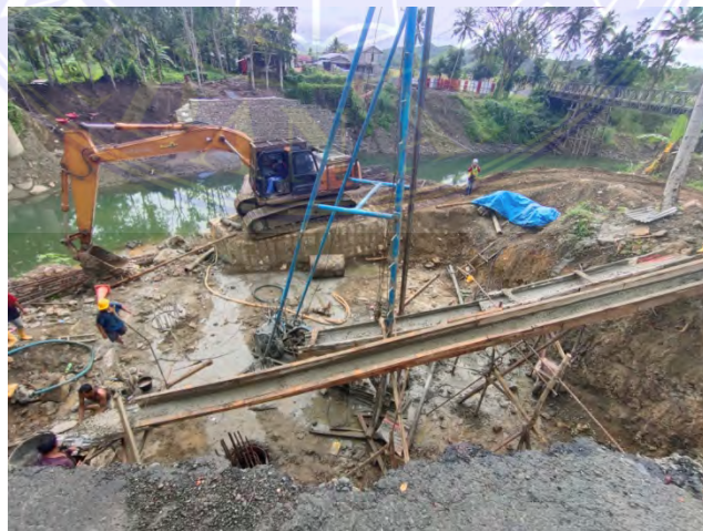
Gambar 4.4. Pengecoran bore pile
