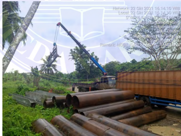
Gambar 3.20. Chasing Bore Pile
