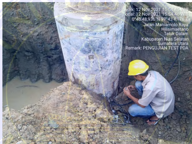
Gambar 5. Pemasangan sensor Accelerometer dan sensor Strain Transducer
