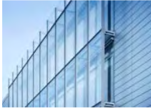
Gambar 62. Sistem Curtain Wall
