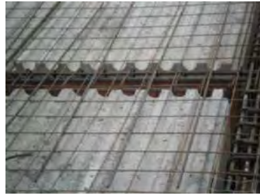
Gambar 2.2 Plat Metode Half Slab Precast
