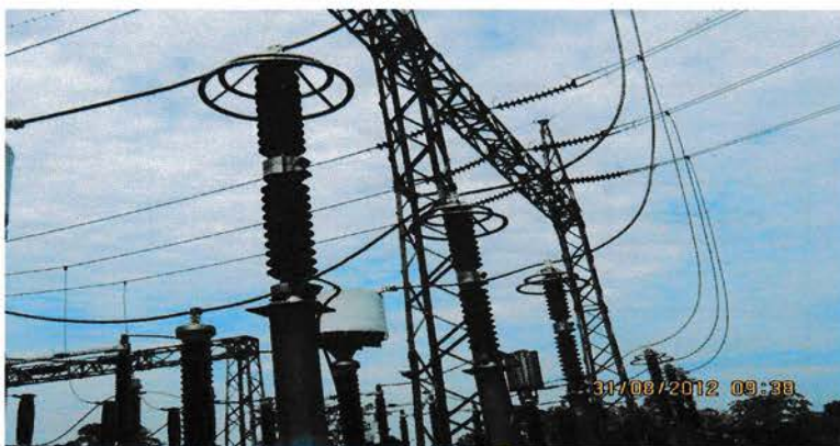
Gambar 2.3 Lightning Arrester GI Namorambe
