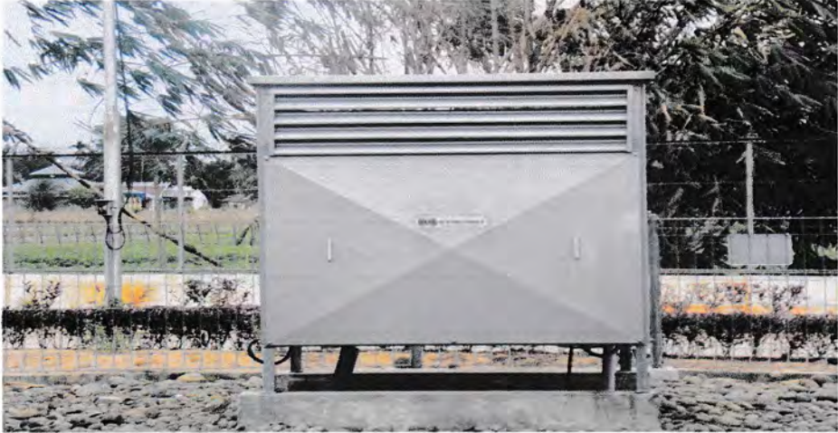
Gambar 2.2 Neutral Grounding Resistance
