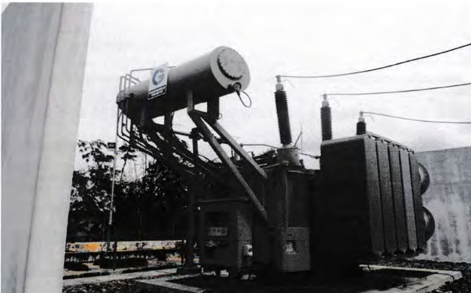
Gambar 2.1 Transformator daya
