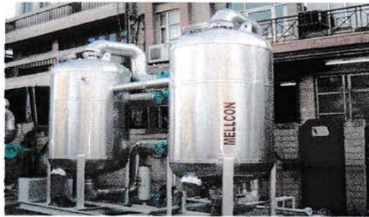
Gambar 3.9. Tank Dryier
