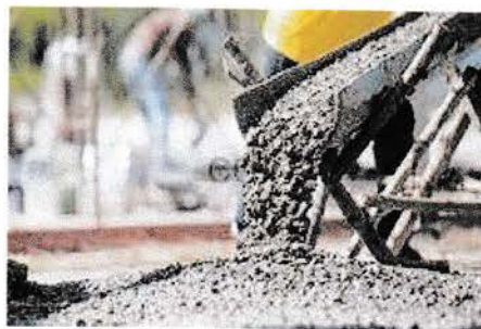
Gambar 3.14 Beton Ready Mix (Sumber : Google search)
