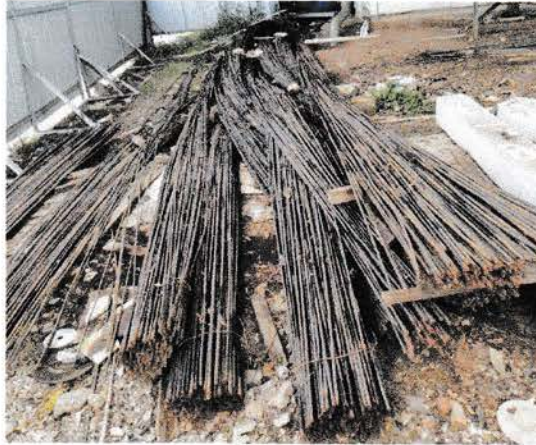
Gambar 3.11 Besi Beton
