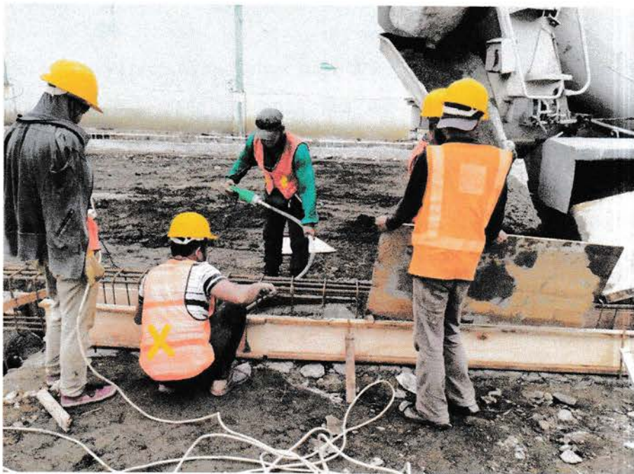
Gambar 4.21 Pengecoran tie beam
