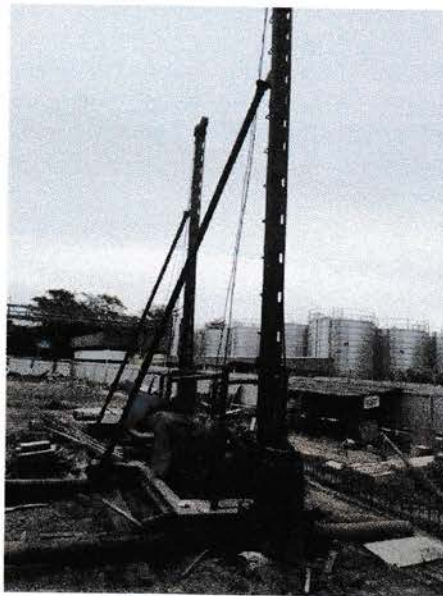
Gambar 3.2 Drop Hammer
