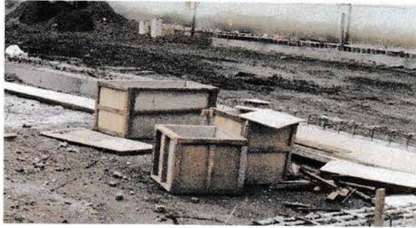
Gambar 4.12 Bekisting PileCap
