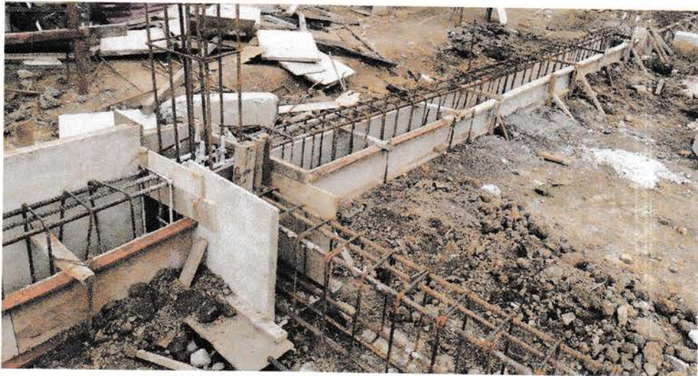
Gambar 4.19 Bekisting Tie Beam
