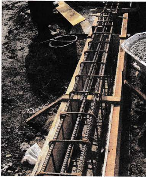
Gambar 4.20 Bekisting Tie Beam
