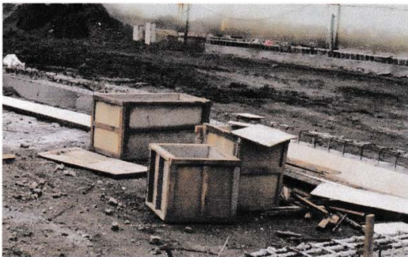
Gambar 4.13 Bekisting PileCap
