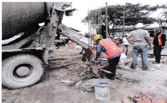
Gambar 3.15 beton ready mix
