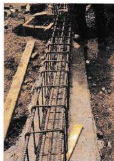
Gambar 4.19 Tulangan Tie Beam
