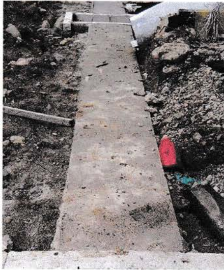
Gambar 4.17 Lantai kerja Tie Beam
