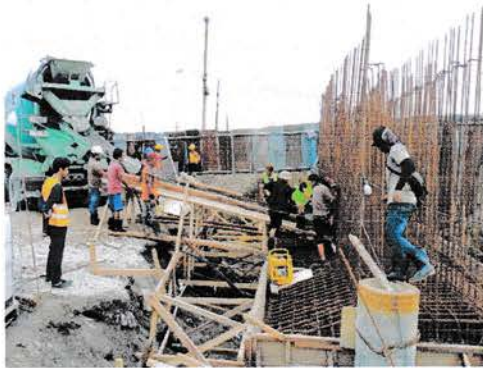
Gambar 3.15 Beton ready mix
