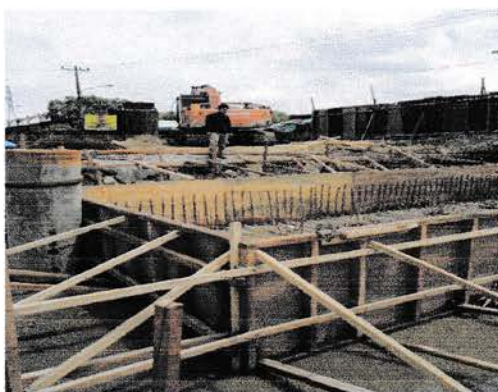
Gambar 3.3 Bekisting
