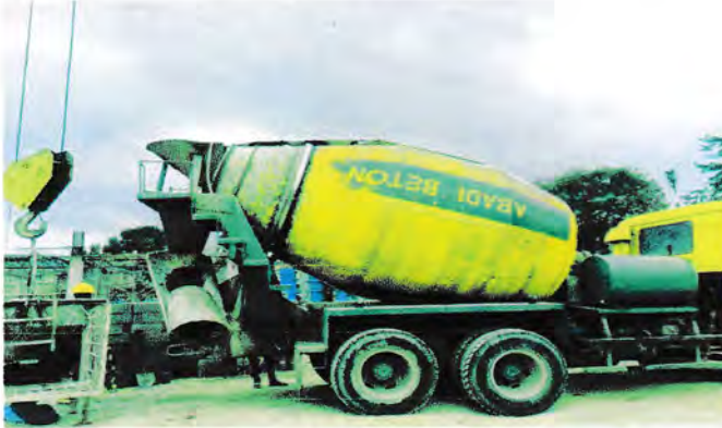
Gambar 3.17 Beton Ready Mix
