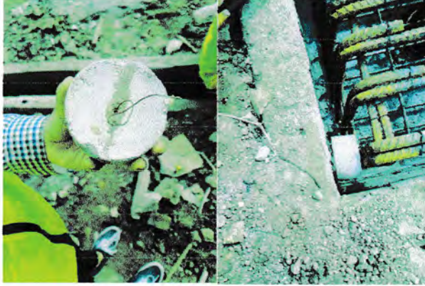
Gambar 3.23 beton deking
