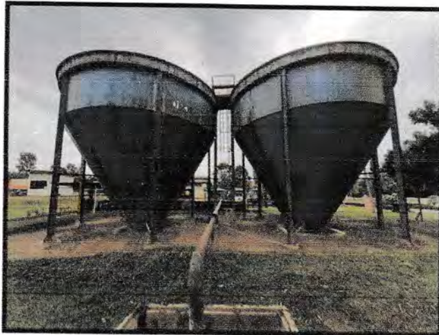
Gambar 3.30 Clarifier Tank
