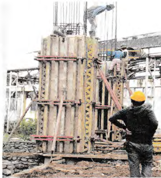
Gambar III.5 Proses Pemasangan Bekisting
