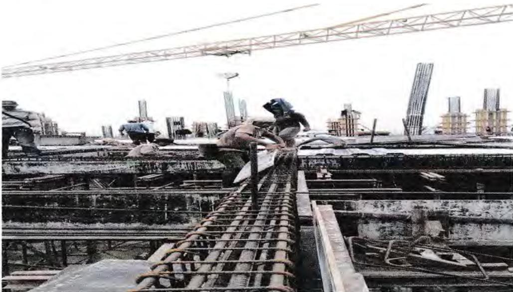
Gambar 3.15 Bekisting balok
