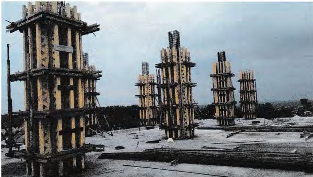
Gambar 3.14 Bekisting kolom
