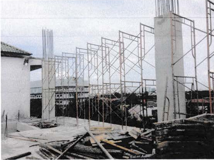
Gambar 3.2.4.Pemasangan Scaffolding
