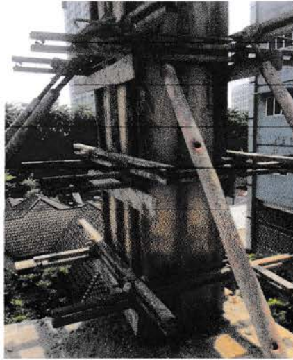
Gambar 3.2.2. Bekisting Kolom
