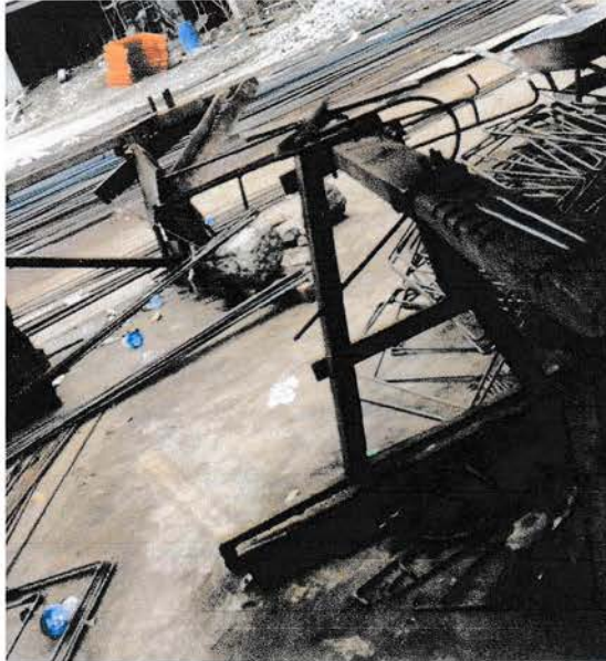
Gambar 3.2. Bar Bending
