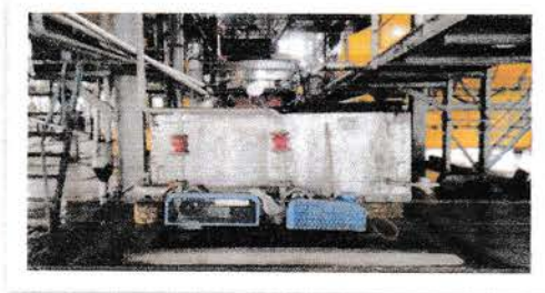
Gambar 5.11. Crude Oil Tank
