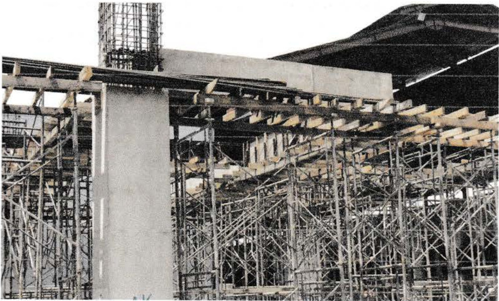
Gambar Scaffolding Sumber : Data Lapangan 2016
