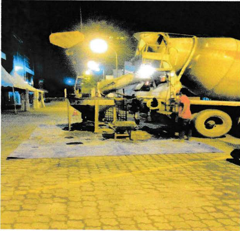
Gambar 3.1 Concrete Mixer (Molen)
