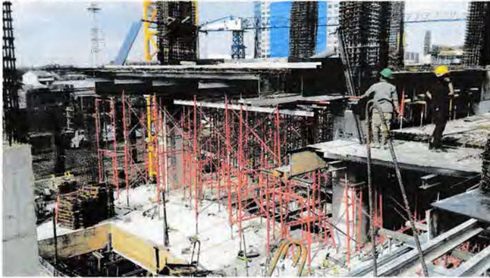
Gambar 4.20 Bekisting Lantai
