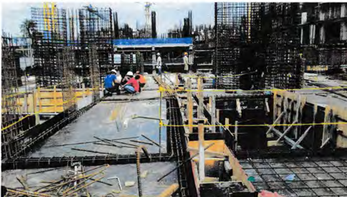
Gambar 4.21 Bekisting Lantai
