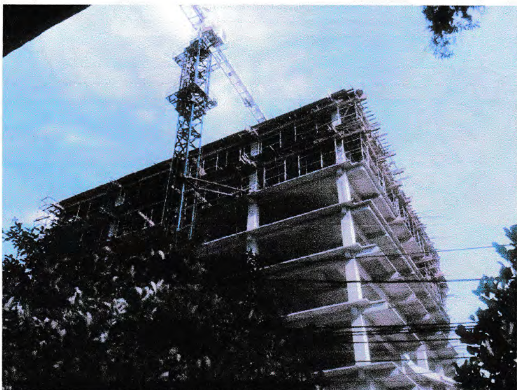
Gambar 46. Tower crane
