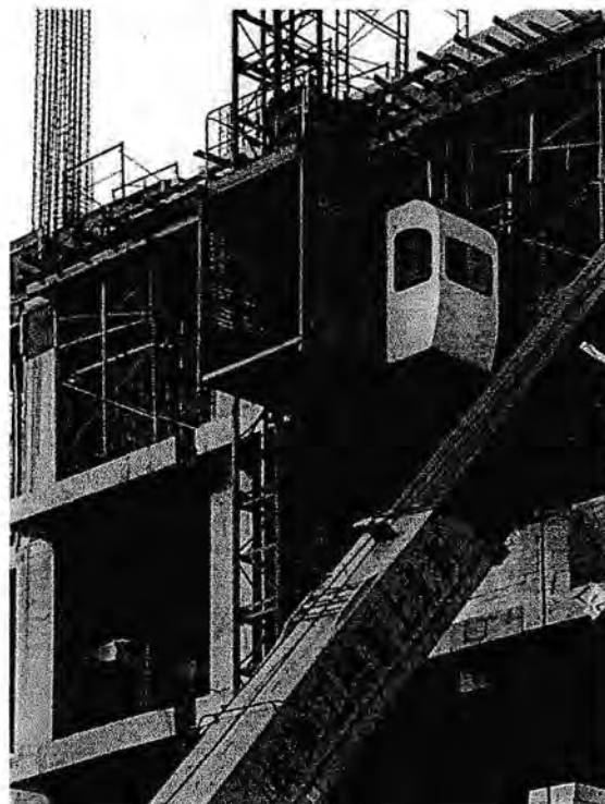
Gambar 3.7 : Passanger Hoist (PH)
