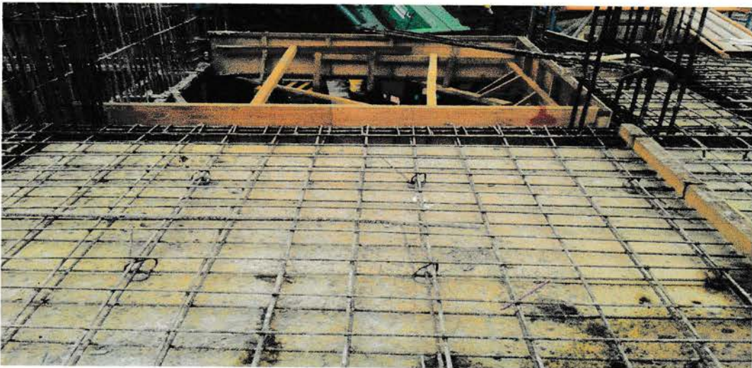
Gambar 3.3. Bekisting plat lantai
