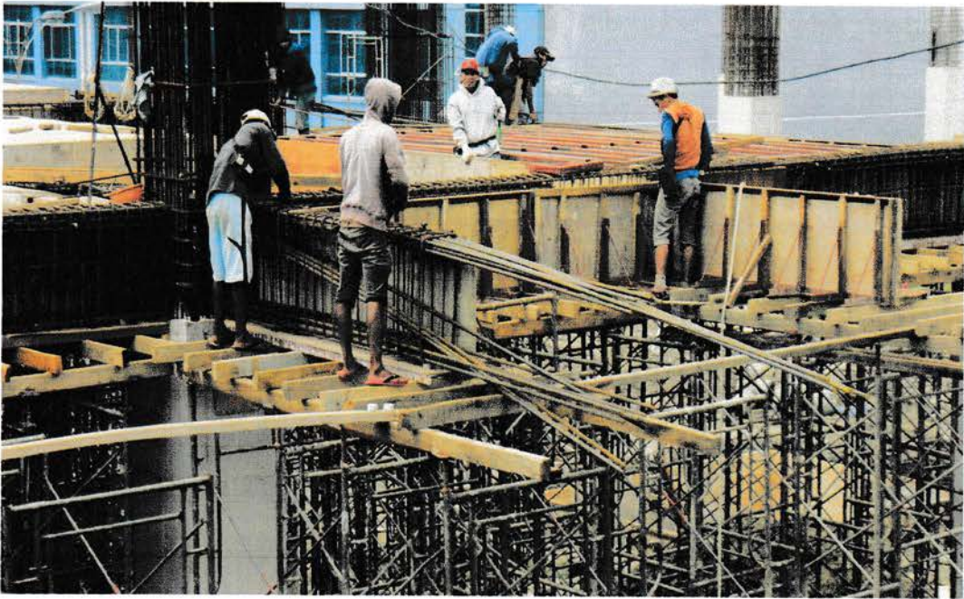
Gambar 3.2. Bekisting balok
