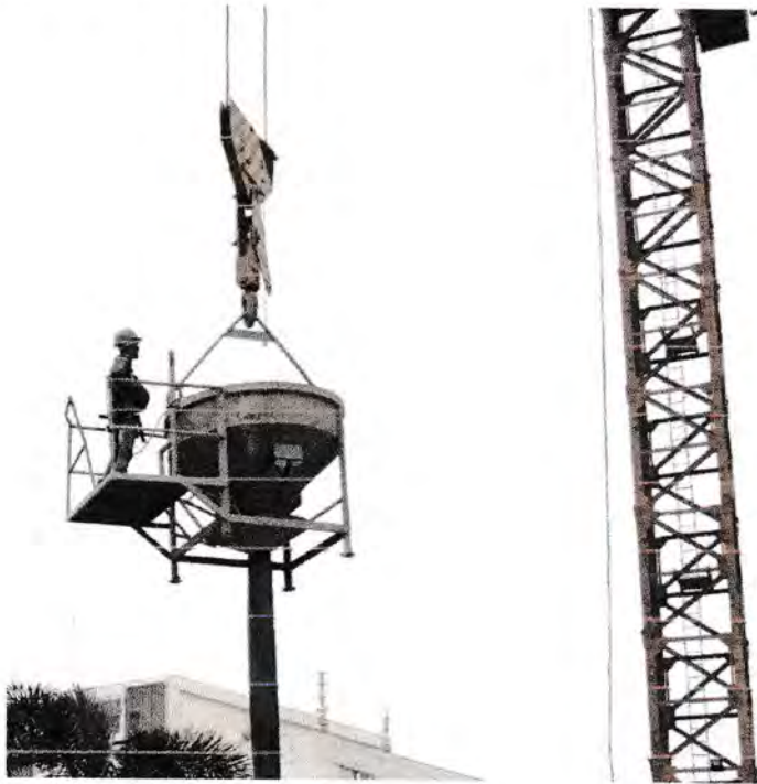
Gambar 3.7 Concrete Bucket dan Pipa Tremie
