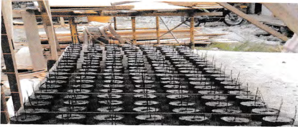
Gambar 3.5 Beton Decking
