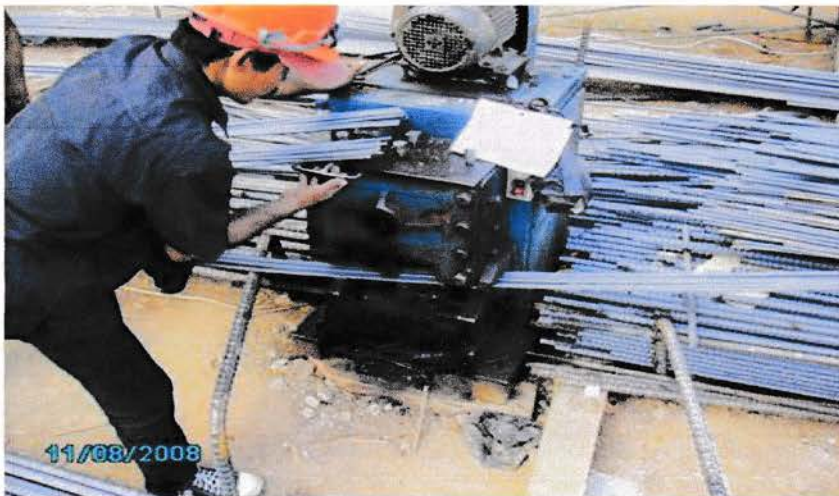
Gambar 2.10.8 Bar cutter
